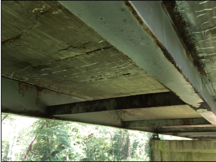
Rust with section loss to lower web and bottom flanges and/or diaphragm connections at all spans. Heavy loss to flange of Diaphragm 1, at Span 1.
