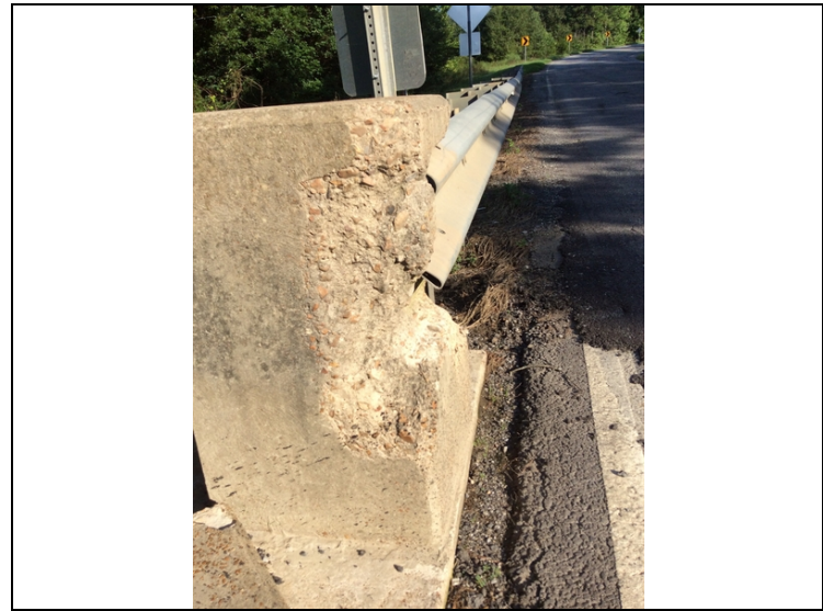
Abutment 2. Large spalls to end posts, some with rebar exposed at Abutments 1 & 2.
