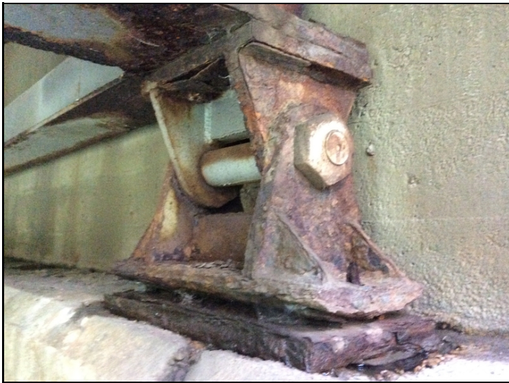
Abutment 1. Typical of section loss to bearing assemblies & missing anchor bolt nuts at Abutments 1 & 2.
