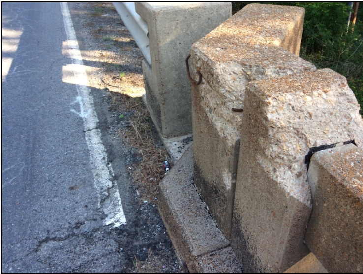
Abutment 2 typical of : Large spalls to end posts, some with rebar exposed at Abutments 1 & 2.
