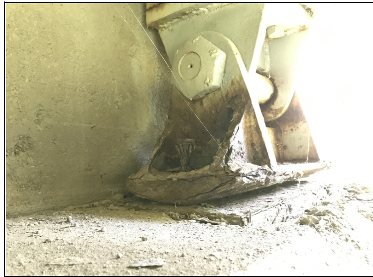
Rust with section loss to bearing assemblies at Abutments 1 & 2 with anchor bolt nuts missing on Bearing 1 at Abutment 1 and on Bearings 1 & 2 at Abutment 2.
