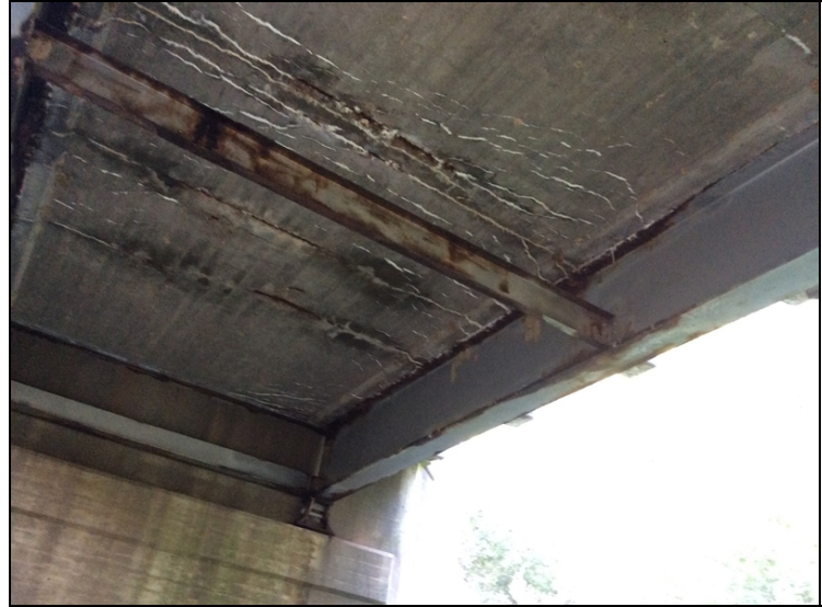
Rust with section loss to lower web & bottom flanges &/or diaphragm connections at all spans. Heavy section loss to flange of Diaphragm's 1 & 3 at Span 1.
