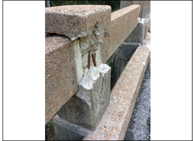
Several concrete posts are spalled and/or cracked at all spans.
