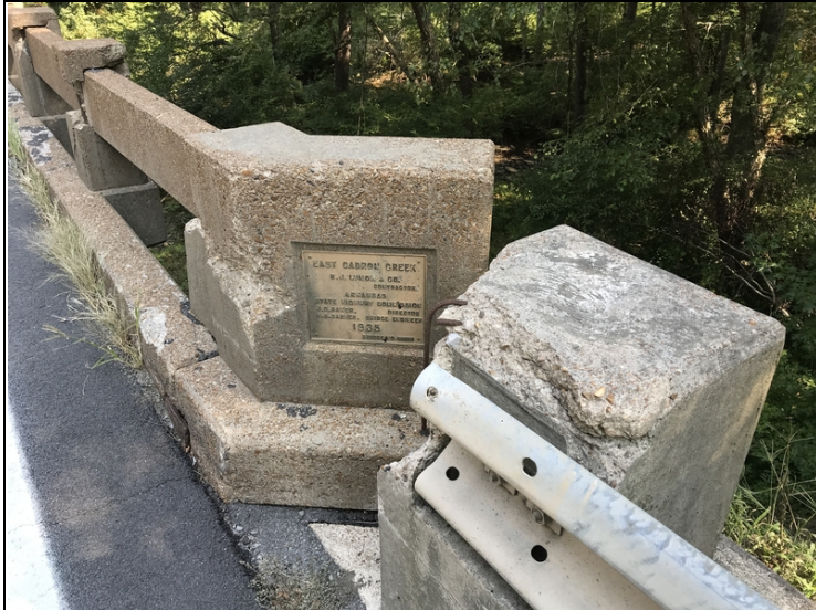
Large spalls to end posts some with rebar exposed at Abutments 1 & 2.
