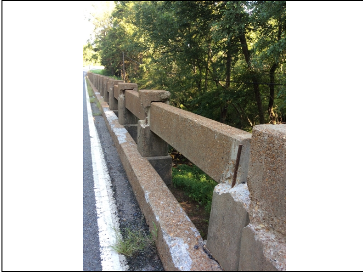
Abutment 1, right side: Several concrete posts are spalled and/or cracked at all spans.
